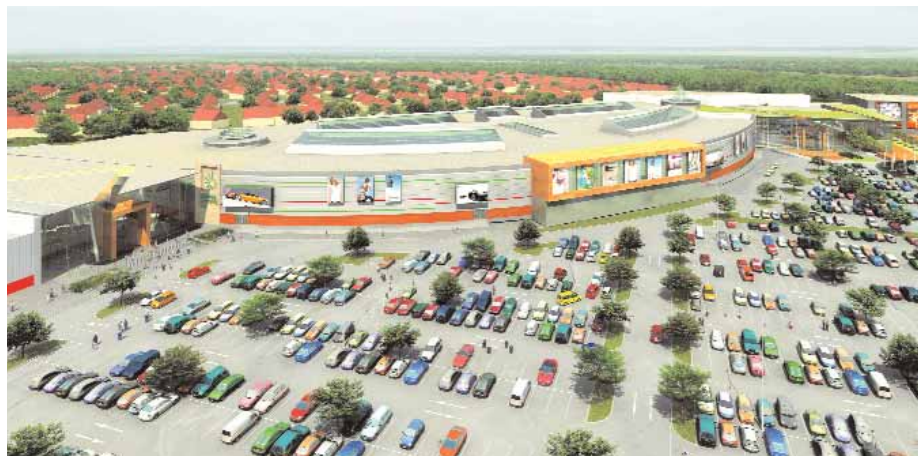
Baneasa Shopping City in Bucharest is the largest mall under construction in Romania.
